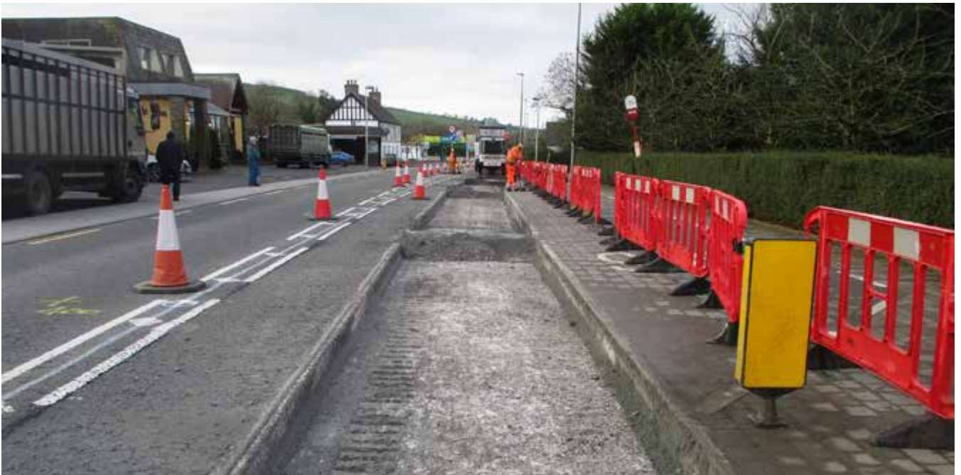
Fig. 1: A planed road surface.
