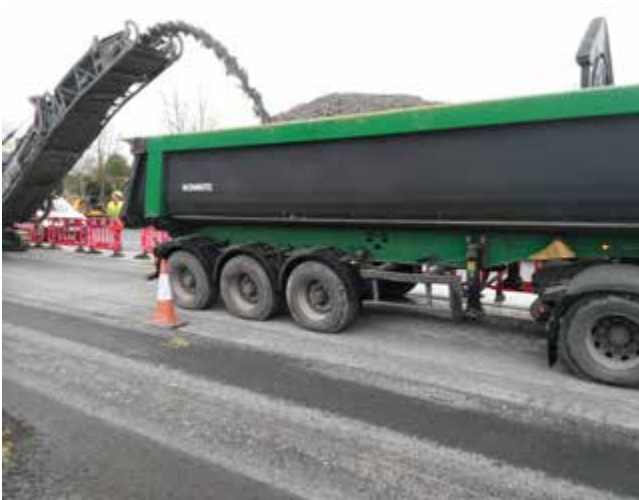
Fig. 2: The milling machine generated the planings
